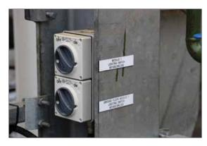
Figure 110: Example of an energy-isolating manually operated disconnect switch with a loop for securing a lockout device (photo courtesy of NZ Steel, Taharoa)
