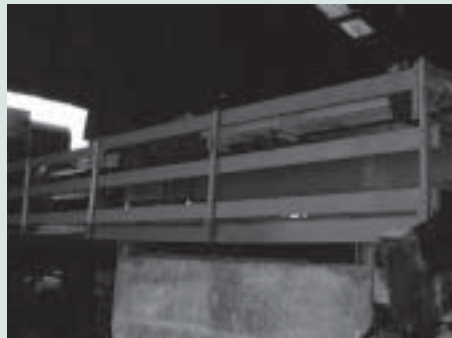
✔ Handrails must be solidly built with mid rail and, where needed, kickboard
