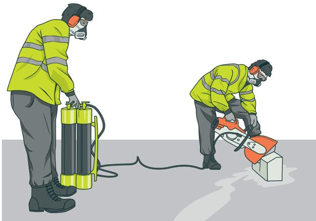
If you do not have a water source at your worksite (for example, you are working in a remote or isolated area) consider using an [on-tool dust extraction system](#) instead of on-tool water suppression. This may be a better option to minimise manual handling that can lead to injuries.
