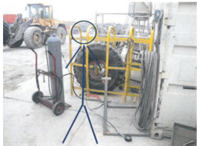
FIGURE 1: The nitrogen cylinder cage and where the worker was standing
