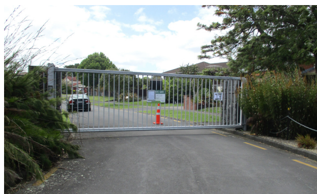
FIGURE 2: Child, represented by cone on other side of gate, was playing near gate housing (left in front of wall). As the gate retracted towards the left side, the child was drawn into gate housing
