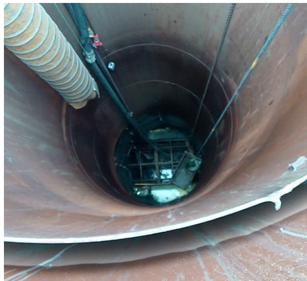
FIGURE 1: Incident Two: View of man cage looking down shaft
