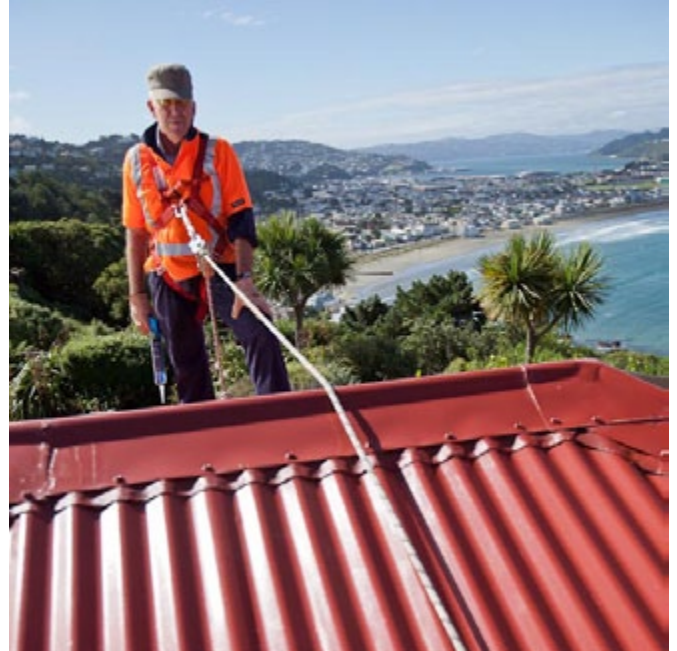
Figure 3: A safety harness and safety line used as a work positioning system.
