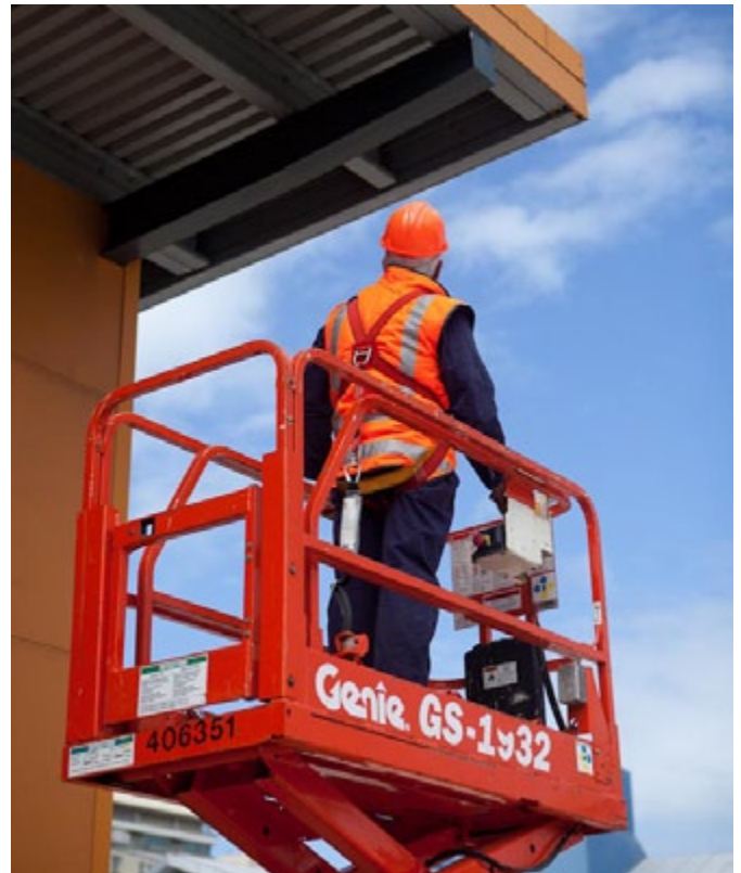
Figure 2: Powered access for inspecting a large fragile roof.
