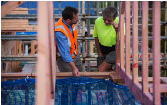
Figure 2: Safety nets installed on a house under construction.
