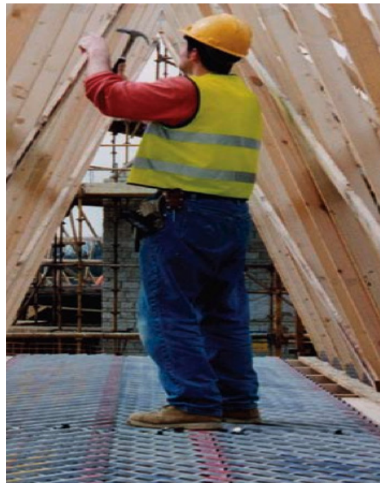
Figure 1: Decking system that provides a working platform in the roof eaves (Image courtesy of Oxford Safety Components Ltd).
